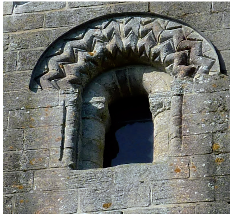
Hedingham: external detail of the great tower parapet
