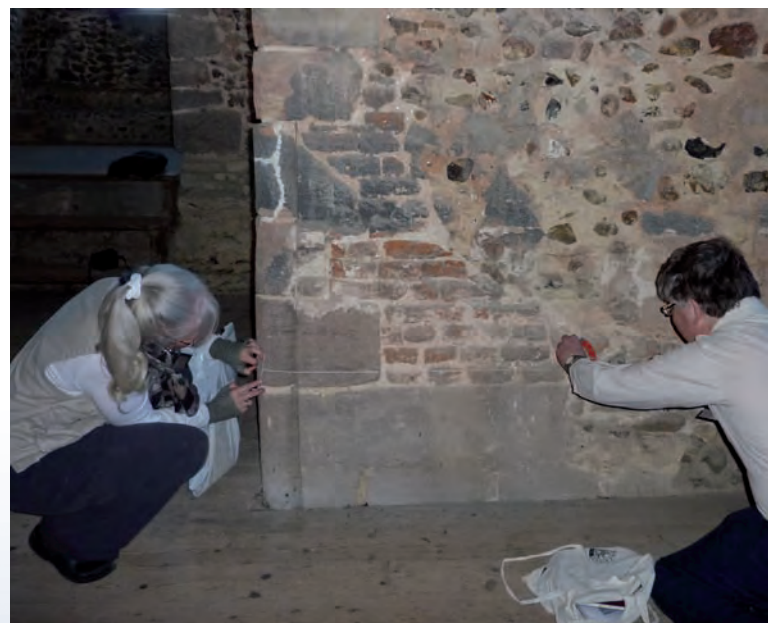
Hedingham: CSG members check out the original roof line
